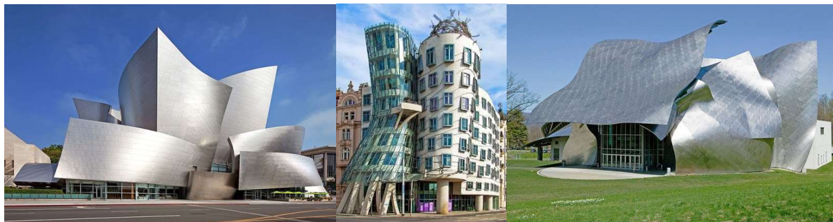
2.8. ábra Frank O. Gehry: Walt Disney Concert Hall, Los Angeles, California; Dancing House, Prague, Czech Republic; Richard B. Fisher Center, Annandale-on-Hudson, New York
