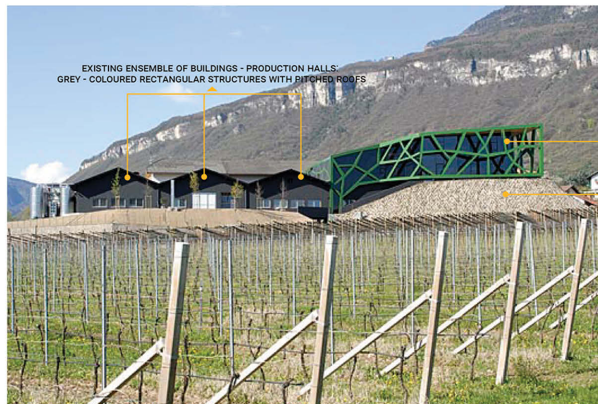
FIG. 4. SIDE VIEW OF THE WINERY'S BUILDINGS, REFLECTING THEIR SCALE, SHAPE AND COLOUR
