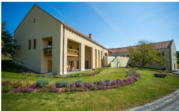
Fig. 4.39, 4.40. General and close up view of the Béres Winery complex (3.000 m 2 | 2006 | WH site | HU)
