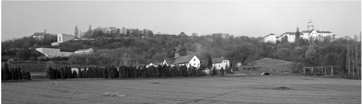
Fig. 4.37. General view of the Abbey Winery Pannonhalma complex and its natural and historical context (1.870 m 2 | 2004 | HU)
