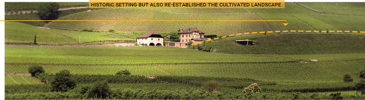
FIG. 5. FRONT VIEW OF THE ESTATE, REFLECTING THE CELLAR'S SHAPE, COLOUR AND THE RELATIONSHIP WITH ITS CONTEXT
