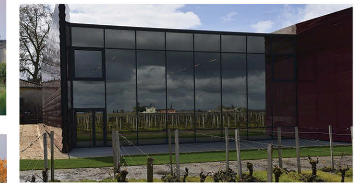
THE USED MATERIALS REFLECT THE SKY, GROUND AND THE ROWS OF VINES, HOST BUILDINGS, LANDSCAPE
