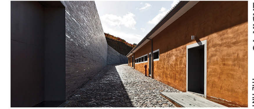
FIG. 4. VIEW OF THE ACCESS BETWEEN EXISTING AND NEW WAREHOUSE
