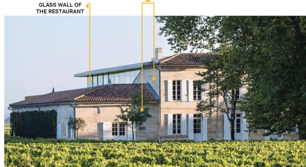
FIG. 5. VIEW OF THE OLD CHÂTEAU AND OLD CELLAR
