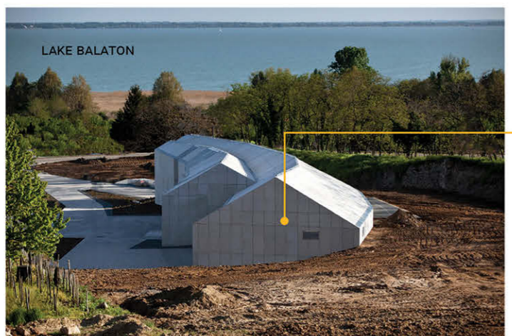
FIG. 4, 5. REAR VIEW OF THE WINERY AND THE CLOSE-UP VIEW OF ITS FACADE, REFLECTING THE USED MATERIALS
