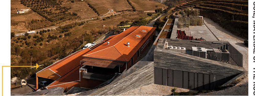
FIG. 5. CLOSE VIEW OF THE NEW FERMENTATION WAREHOUSE
