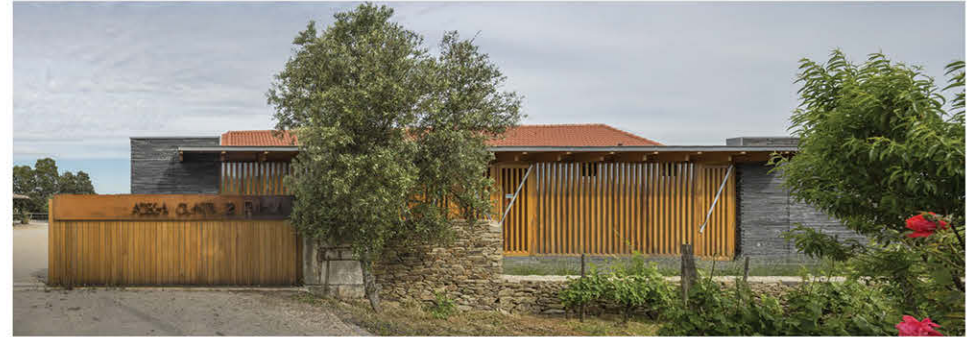
FIG. 7. SIDE VIEW OF THE EXTENTION, REFLECTING THE USED MATERIAL
