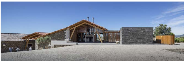
Fig. 4.43, 4.44. General view of the Quinta da Faísca and its cultural context (2013 | WH site | PT)
